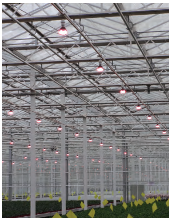
Figure 1. Several factors influence the efficacy of photoperiodic lighting fixtures, including tolerance to greenhouse conditions and the method, intensity, and spectrum of lighting.
